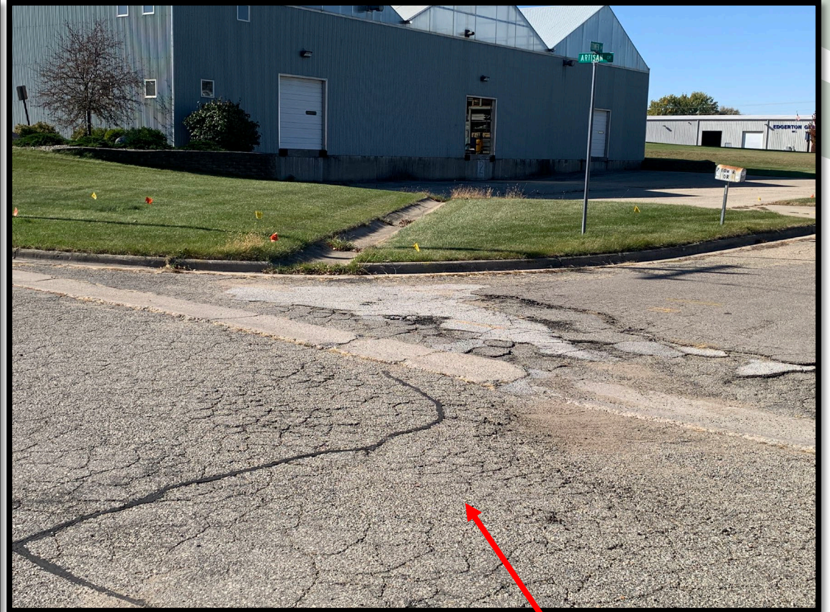
Alligator Cracking
